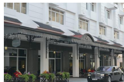
PARADISE SUITES HOTEL, HALONG BAY
